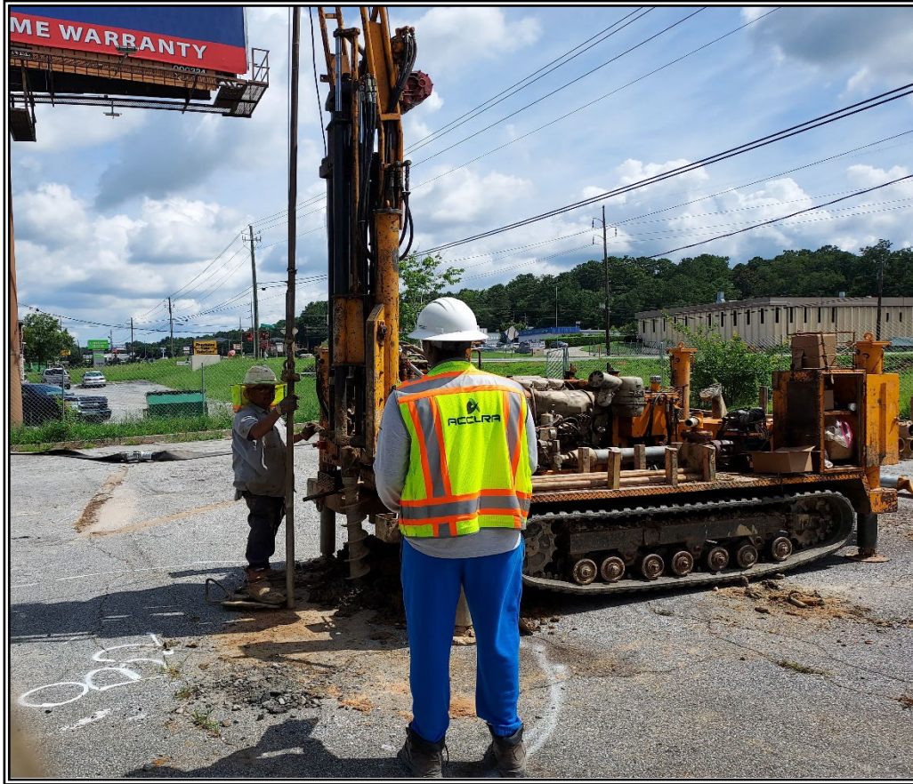
Showing of borehole operation near sinkhole.
