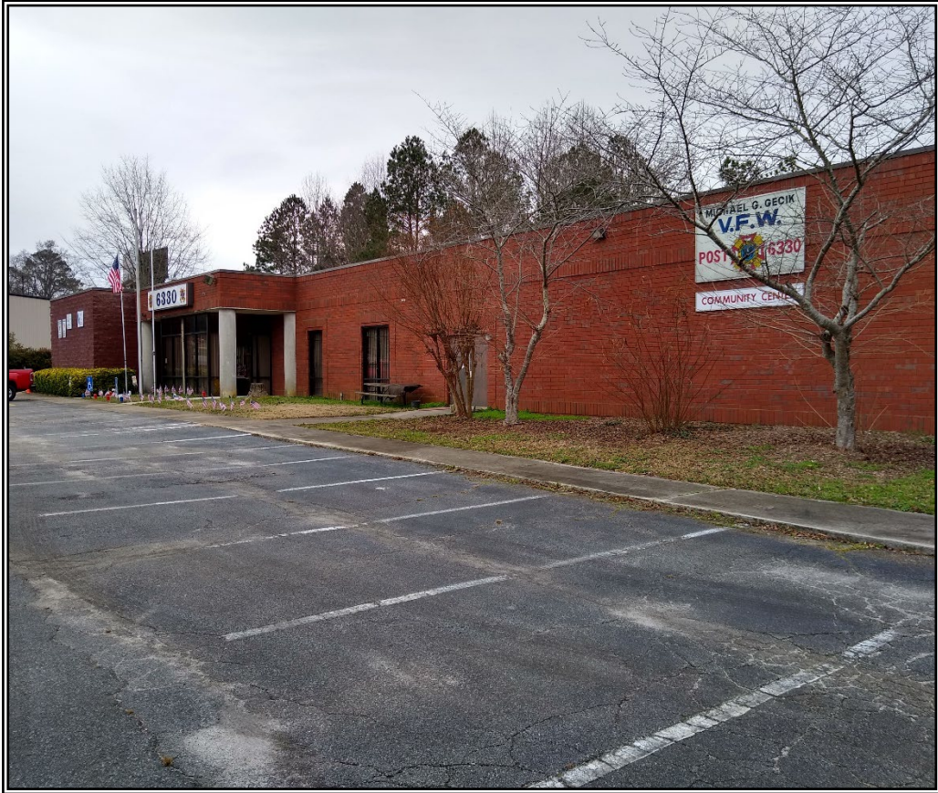
Front view of Veterans community center building and parking lot.
