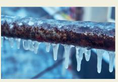
Insulate pipes in unheated areas like basements, attics, and garages to prevent freezing.
