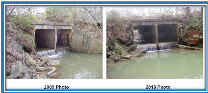
Photo: Creek Culvert Repairs – Rock Cut Road
