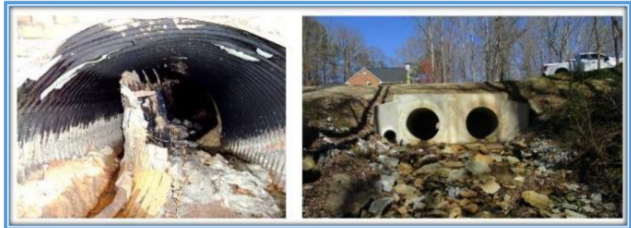
Before and after photographs of a culvert renewal.
