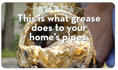
Fats, oils and grease clog sewer lines and cause blockages (like in the photo above) resulting in costly sewer backups. Instead of pouring cooking grease down the sink drain or toilet, let it cool. Then, pour it into a plastic container or metal can with a lid. Once the container is full, just toss it in your kitchen garbage.
