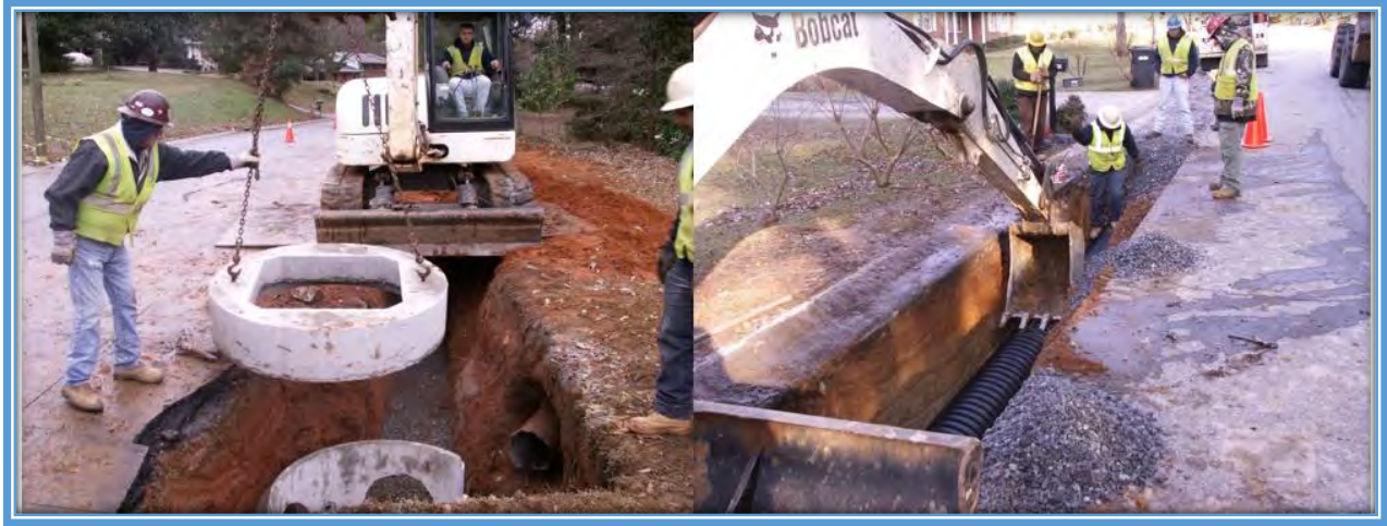
Before and after photographs of a culvert renewal.
