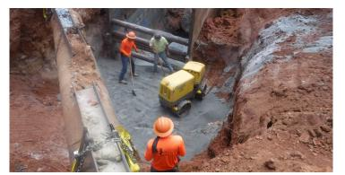
160' long. The culvert eroded and separated at several joints. The culvert was over 20' deep under the roadway. Plus, two of our potable (drinking) water mains were on either side of the roadway, along with a gas main. This project also included another storm drain system from a nearby subdivision that needed to be replaced.
