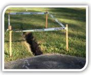
Jackson Estates Subdivision. In addition to the forming sinkhole, we found the culvert was severely corroded, and extreme sediment buildup at the discharge end of the pipe.
