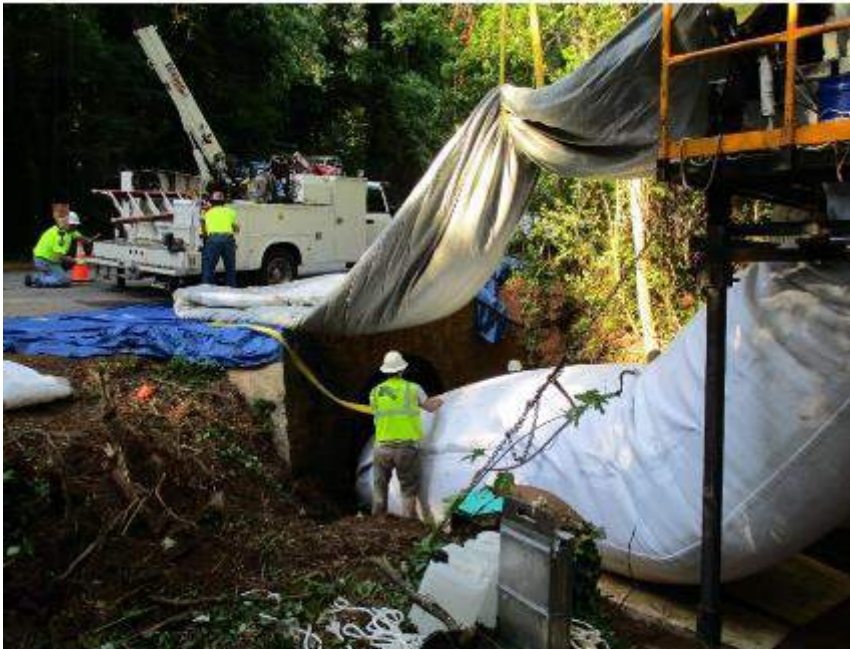
SW004 – STORMWATER CURED-IN-PLACE PIPE (CIPP) – [SMP 214]
